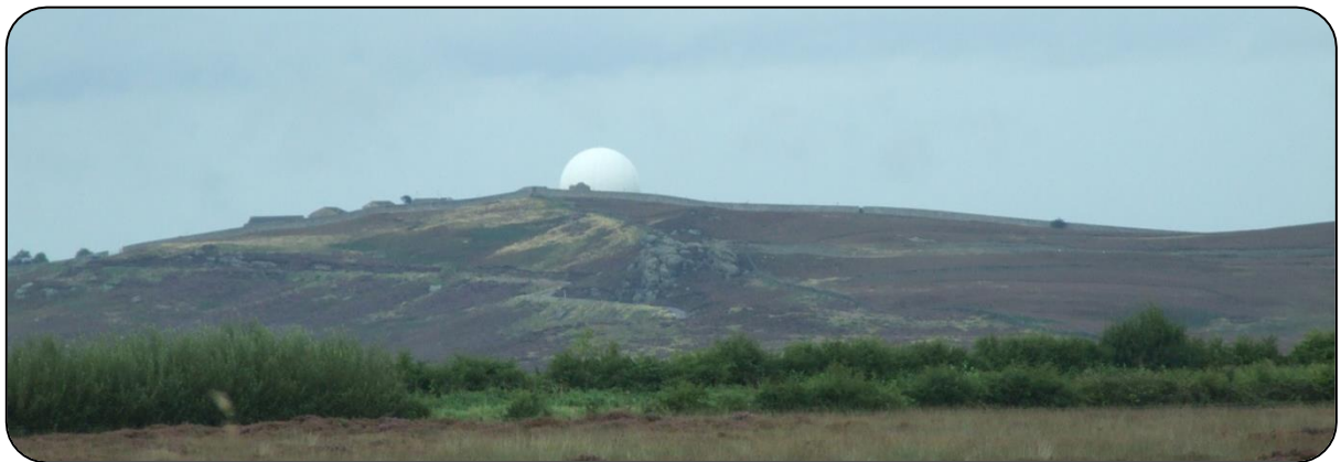
Figure 2: RAF Brizlee Wood Radar
